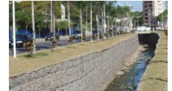
Longitudinal protection on major river
