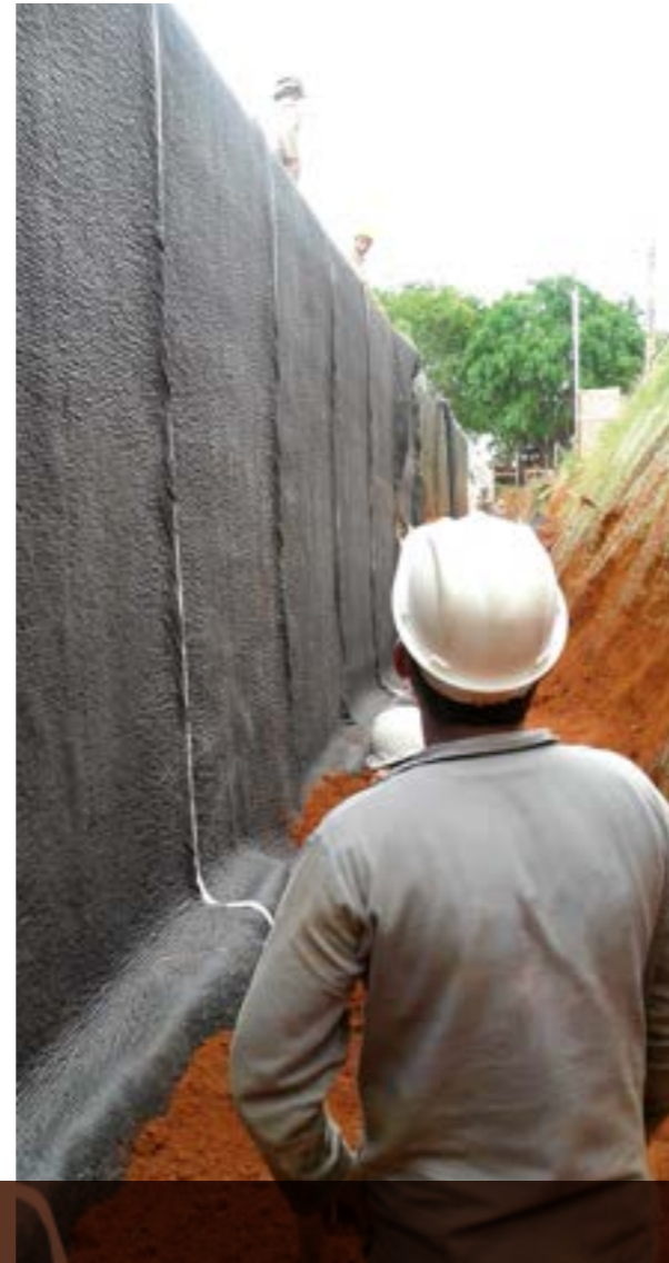
Railway track drainage
